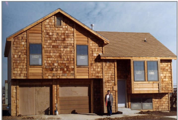
Mary in front of their under construction home in Lawrence.
