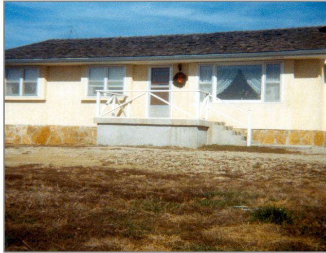
Marshes' home in December of 1981. In 1977 Rex is starting to put the stucco on the house.
