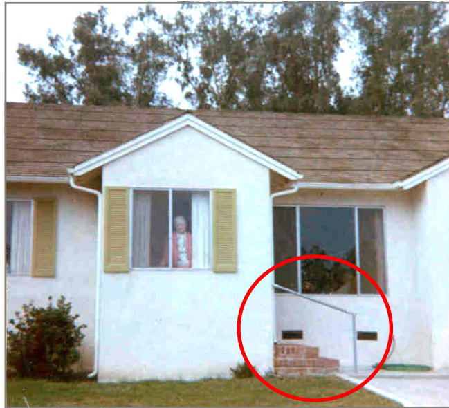
Handrail Rex installed is circled above.
