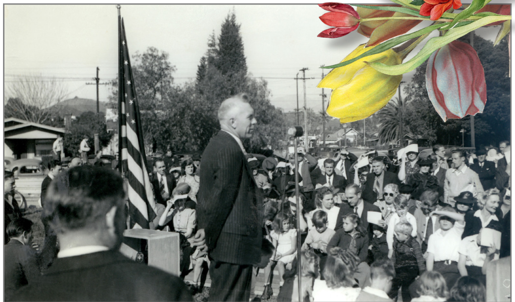
Bishop Al Hoglund at the ground breaking of the Garvanza Chapel in 1941.
