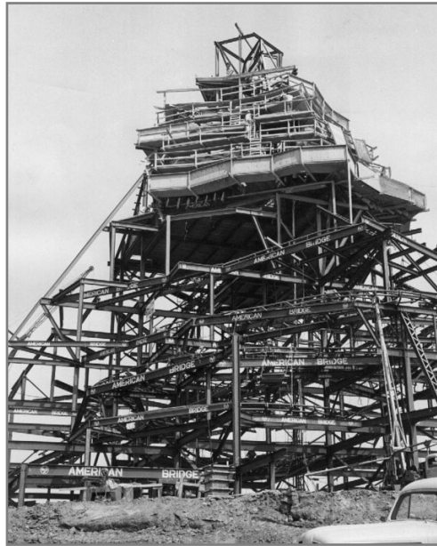
The Matterhorn at Disneyland as Elvie and Lou would have seen it. The ride under construction in March of 1959, it opened on June 14, 1959.
