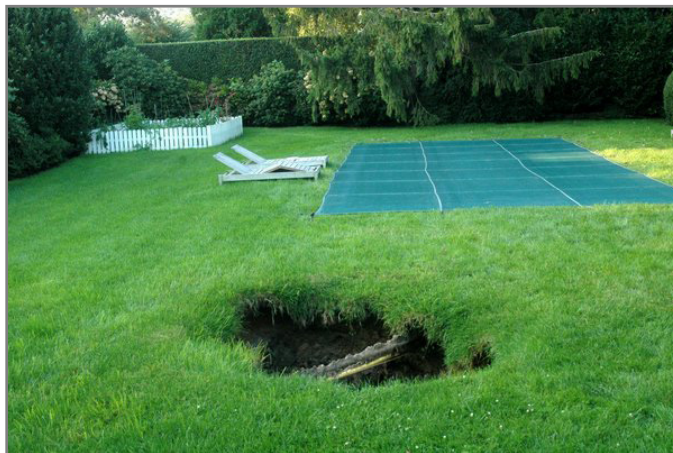
Old block style cesspool collapses.
